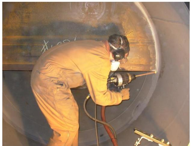
Figure 7: Robotic application of the Hastelloy C- type HVOF coating onto inner surface of the outlet channel of the sulfur condenser with the AK-07 gun (a) and hand-held application with the AK-06 gun over the welds after installation of the de-mister structure (b)
